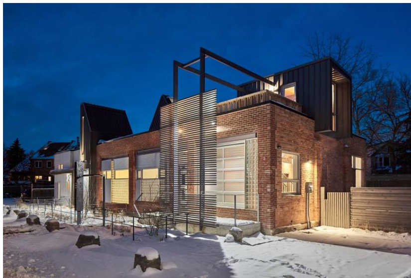
The original building, top, and the 'Mr. White' townhouse after the renovations.
