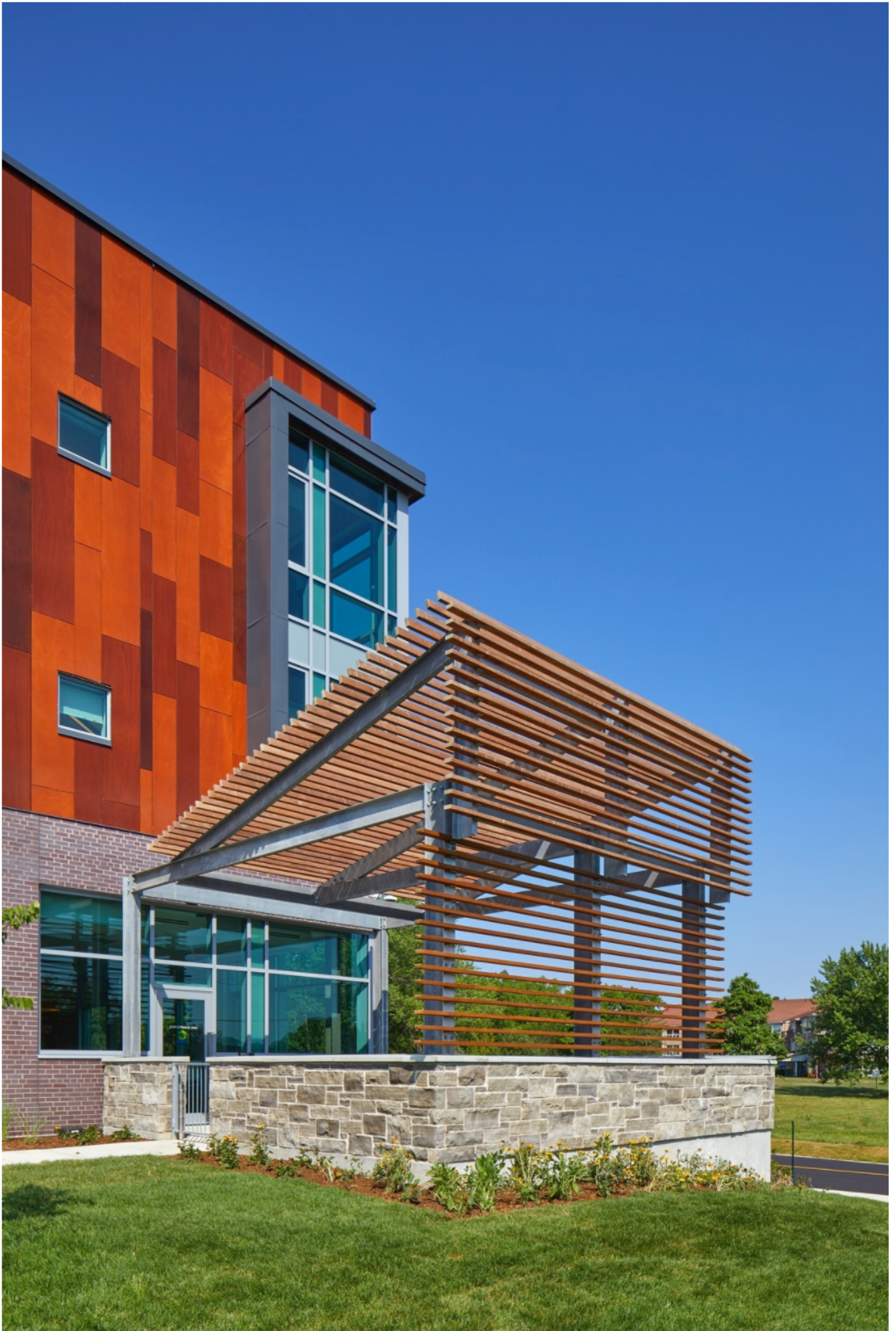
Extensive new trees surround the CAP, including along the upgraded Chippewa Street and between the building and the parking area, helping to soften the transition from landscaped to hard surfaces. Photo Credit: Tom Arban
