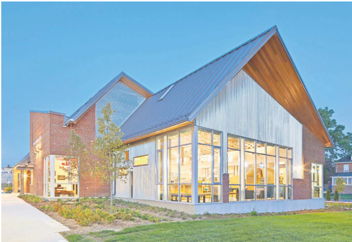
The materials used for the Haldimand County Library and Heritage Centre echo those of nearby buildings. The brick is reminiscent of that used on a law office across the street and on retail buildings nearby, while the corrugated metal siding references the grain silos, barns and storage buildings dotting the landscape. PHOTOS BY TOM ARBAN
