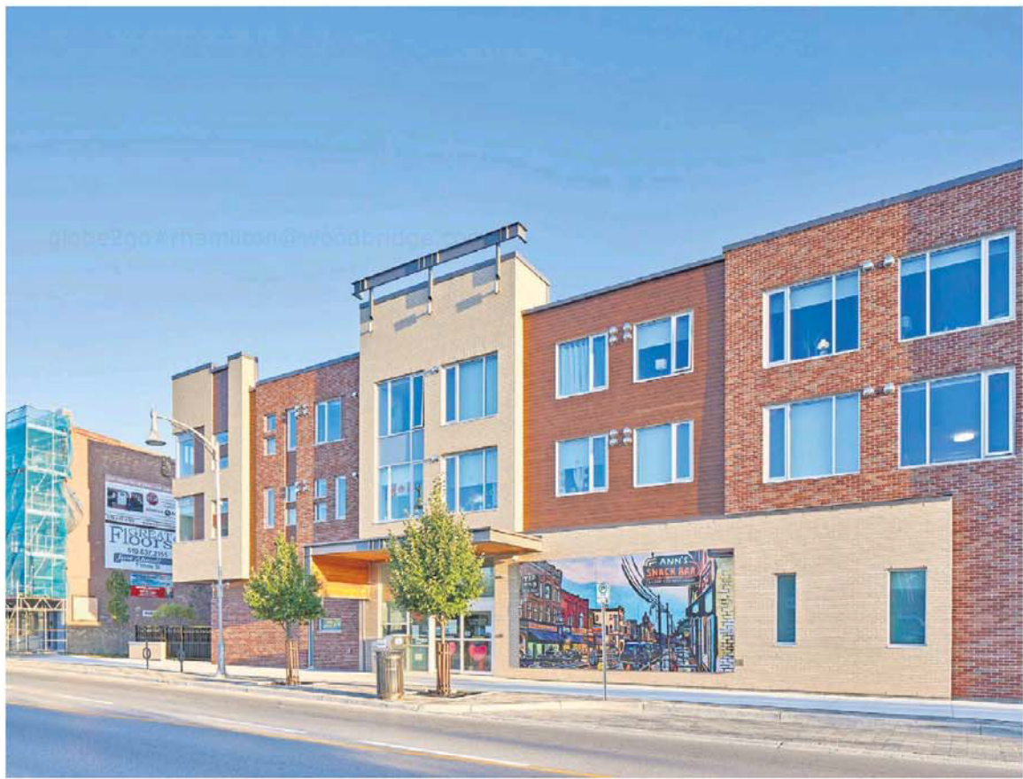
Hamilton-based Thier + Curran Architects designed this three-storey brick building at 230 Talbot St. in St. Thomas, Ont. TOM ARBAN
