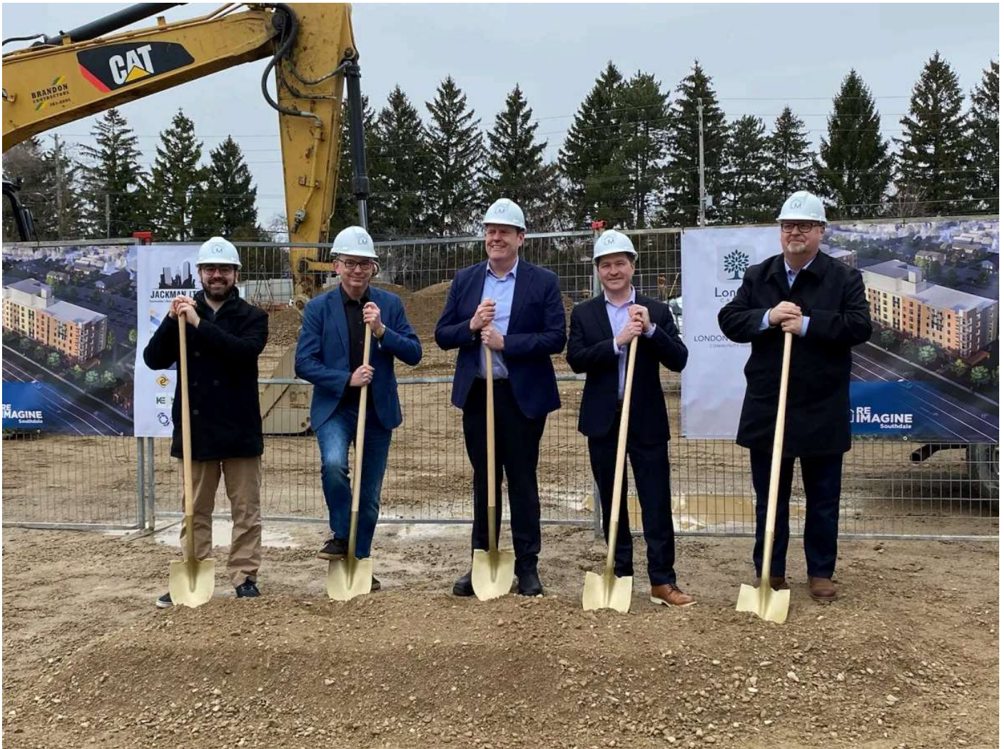
Officials from both the city and LMCH were present Wednesday, March 6, to break ground on phase one of Reimagine Southdale. Ben Harrietha/980 CFPL
